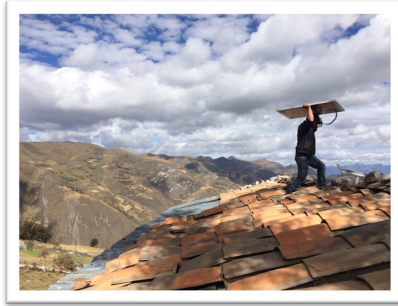
(Technician from a local NGO installing a solar home system. Province of Santa Cruz, Region of Cajamarca, Peru. Photo by author.)
